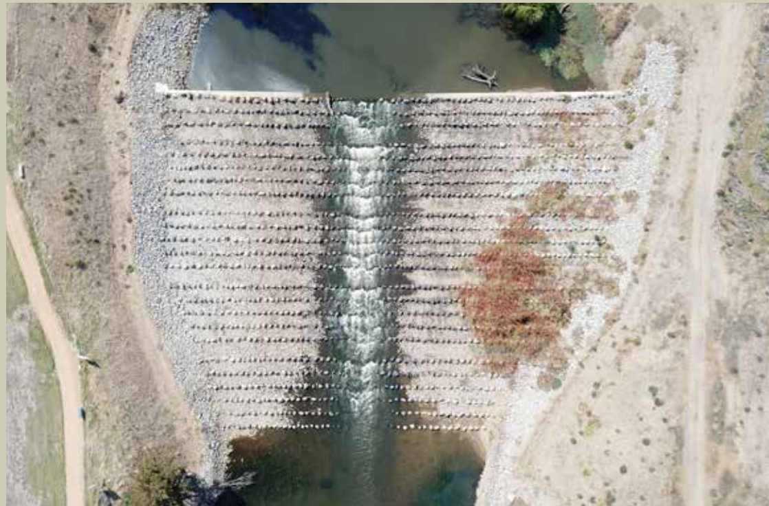
Upgraded South Dubbo Weir, including rock ramp and fishway.
