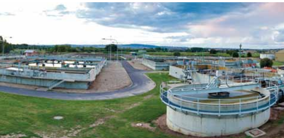
BELOW Wastewater Treatment Works, Bathurst
